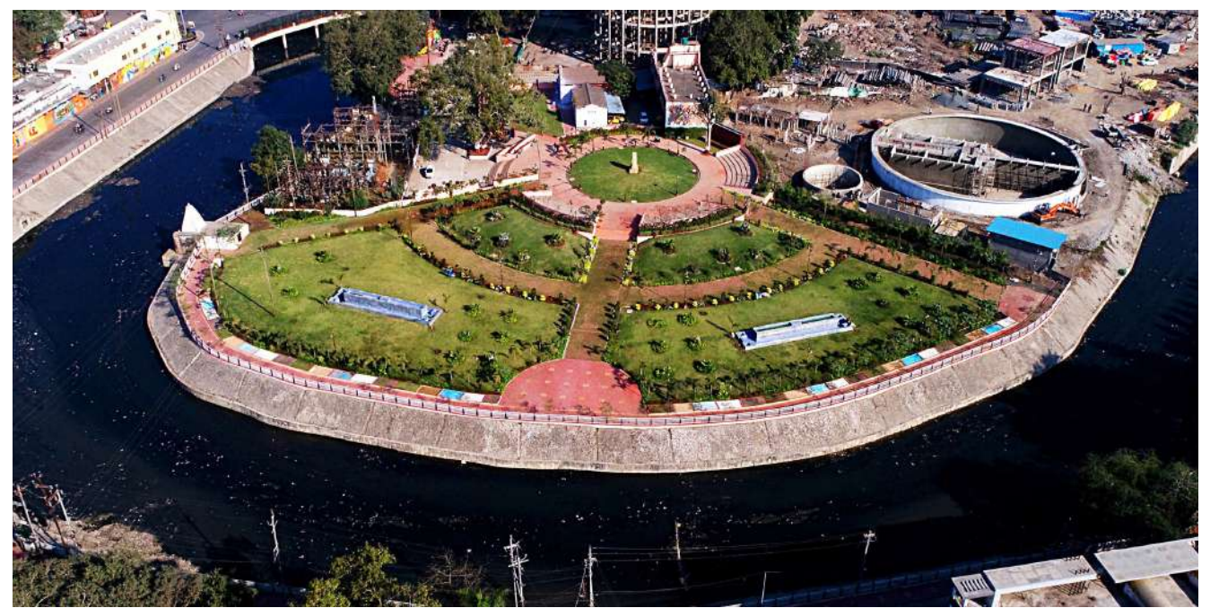
Indore Smart City river front development. Recreational open spaces along the Kahn River (25 OCT, 2022)
